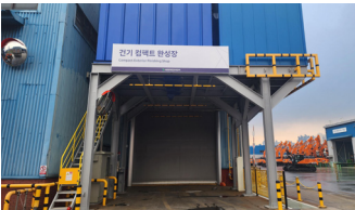
Incheon Plant RTO
