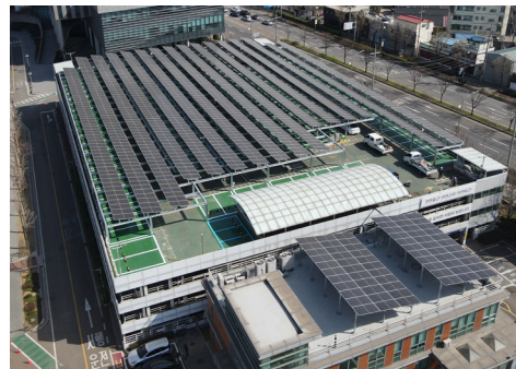
Solar Power Generation Facility in Incheon Operations
